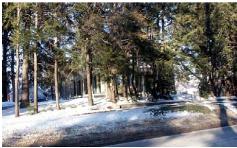
Existing conditions image of The Homestead
