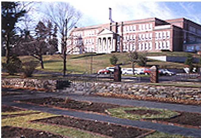
Under Restoration – Fall 1999
