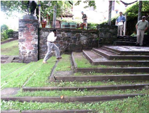
Existing conditions, Aug. 30, 2006
