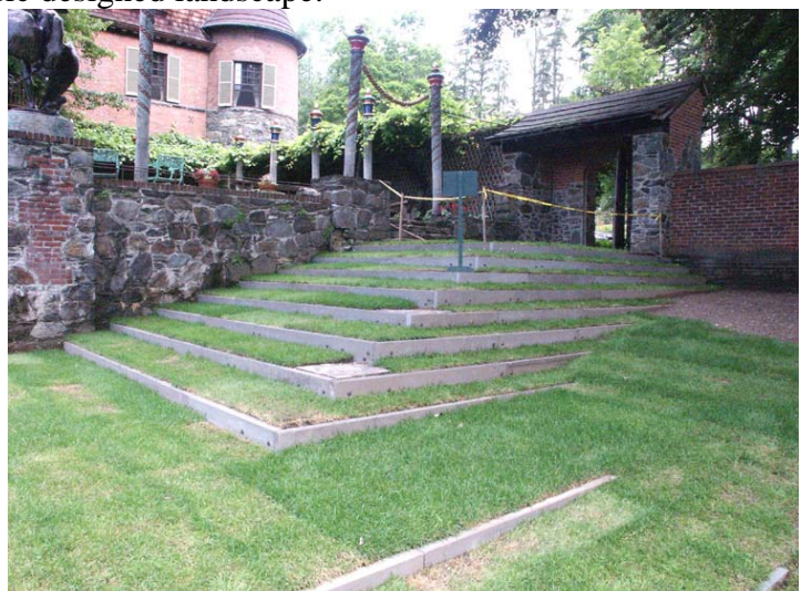
Restoration complete, July 20, 2007
