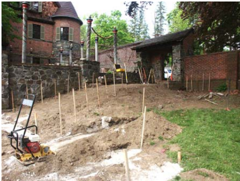
During restoration, May 2007
