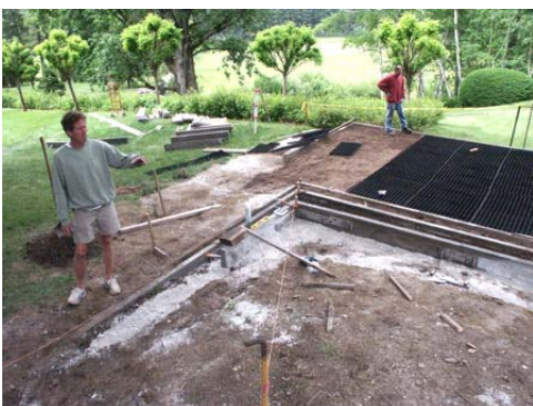
During restoration, June 14, 2007
